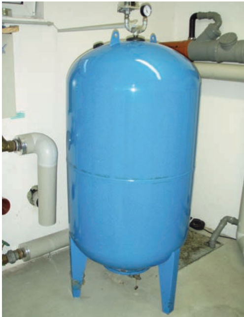
Abb. 13: Membrankessel, © AGES
